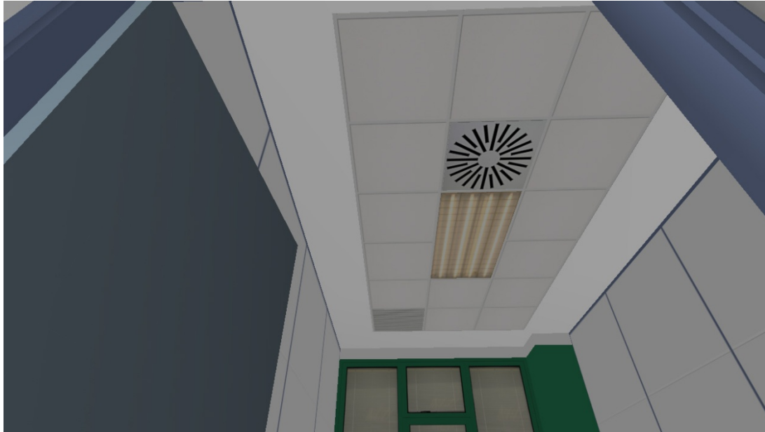
Fig. 23. Paneled office ceiling with fluorescent lamps and air conditioning diffuser
