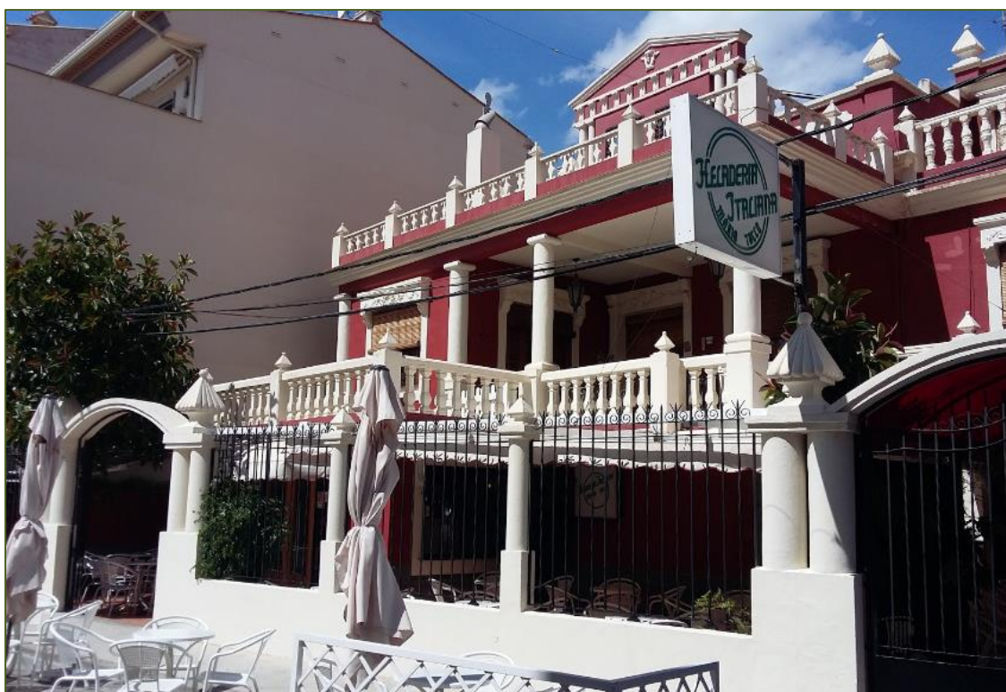
Figure 5: Facade of the store of Altura
