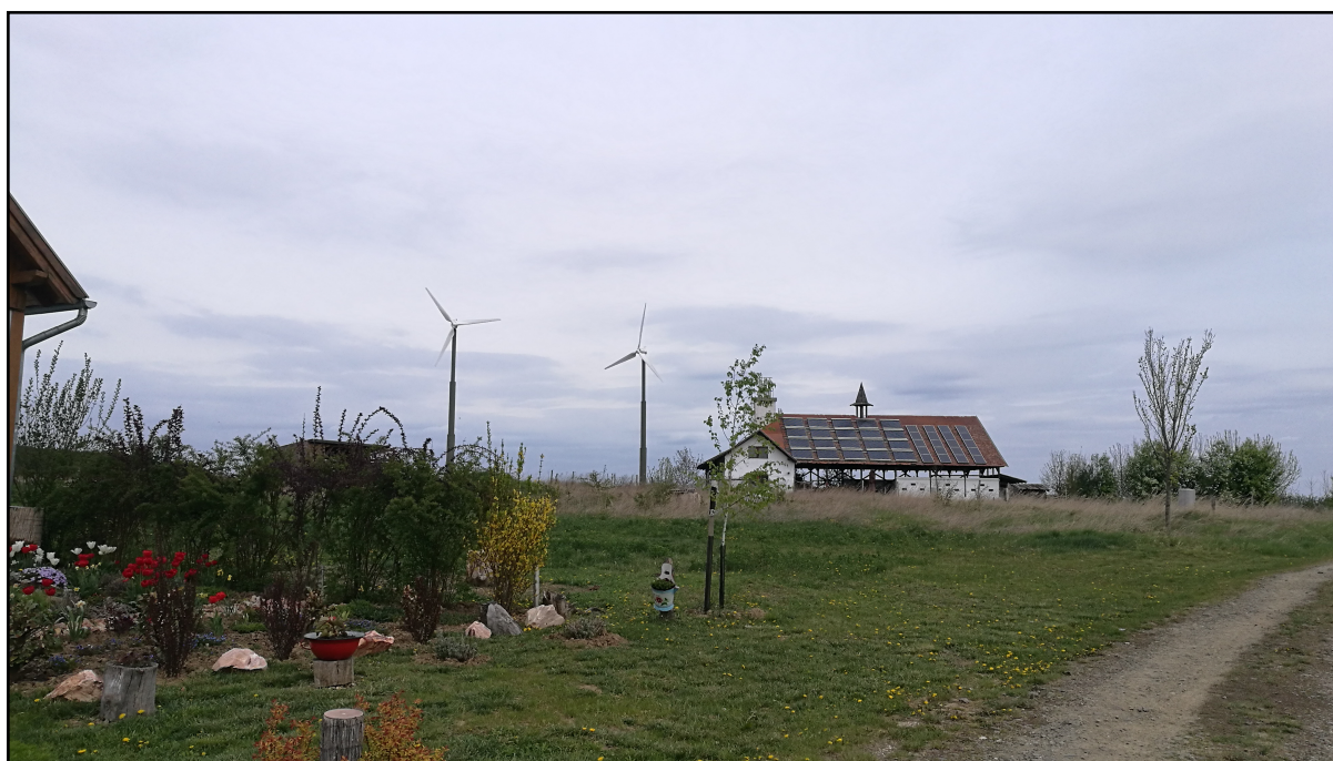
Figure 7 - Photograph of a wind turbine type from the eco-village
