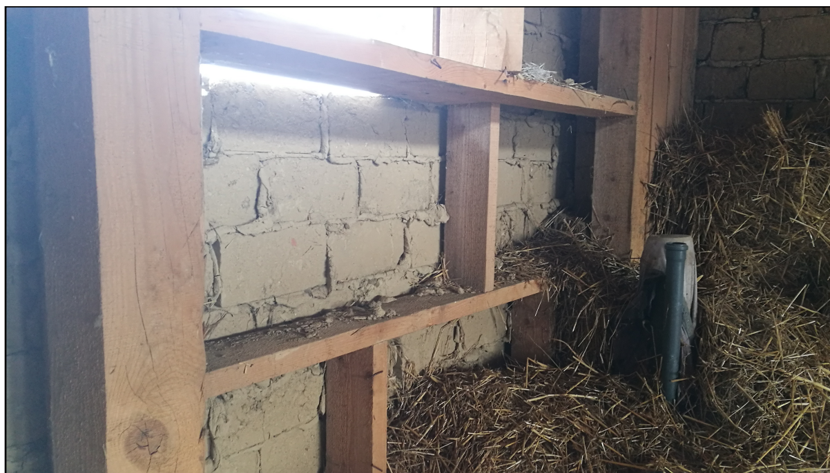
Figure 13 - Photography of the building wall structure
