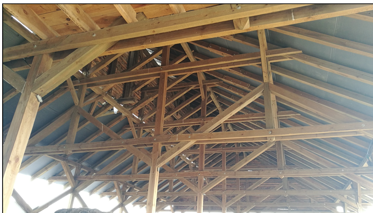
Figure 8 - Photograph of the wooden structure of a common eco-village building
