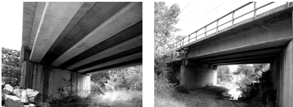
Figure 1: Railway bridge in High Speed line composed by short simply supported bays
