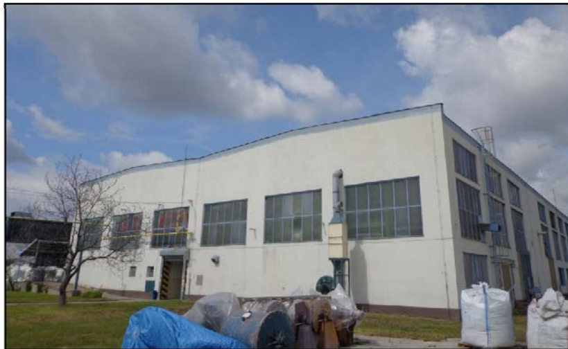
Figure 5.1 Building chosen for the PV installation
