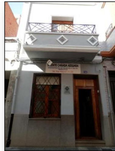
Imag.1 : Fachada principal
