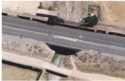
Figure 2. HSL bridge under study (38°43'33.06"N 4°5'20.05"W).
