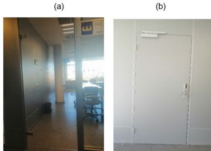
Figure 4.2: (a) Glass door with high contrast. (b) Door and wall share the same color, making it challenging to distinguish the door frame.
