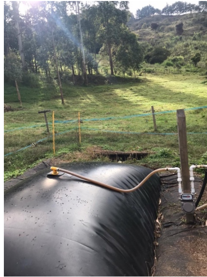
Figure 1: Psychrophilic tubular low-cost digester implemented in Colombia.
