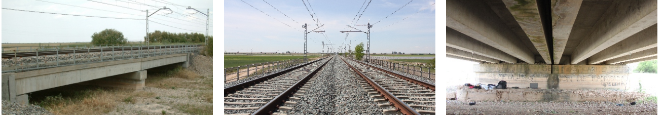
Figure 12: Bridge over the Old Guadiana watercourse images.
