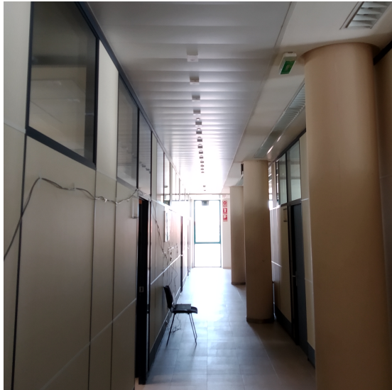
Fig. 2. Beacons deployed on the ceiling of the corridor.
