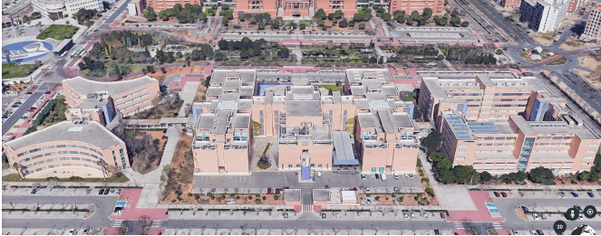
Fig. 1: 3D areal view, from Google Earth, of the three buildings considered in this section’s experiments. From left to right, the buildings are identified as TI, TD and TC.
