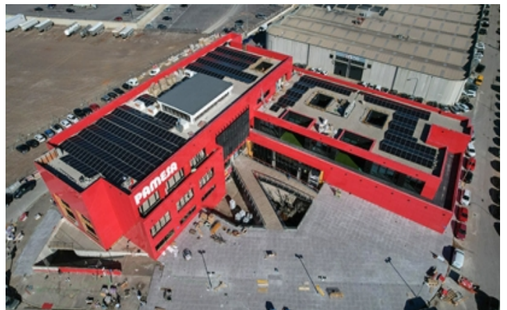
Image 38: Solar panels new office
