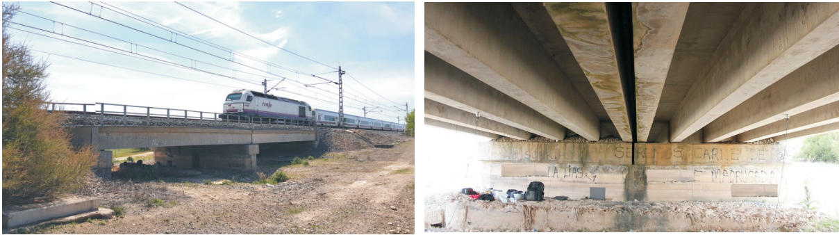
Figure 12. Old Guadiana River Bridge.
