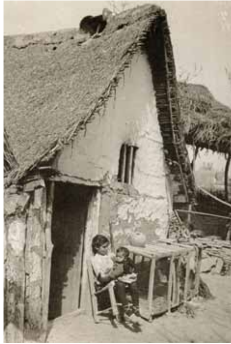
[Fig. 6] Picture from a Spanish traditional construction, 1935.
