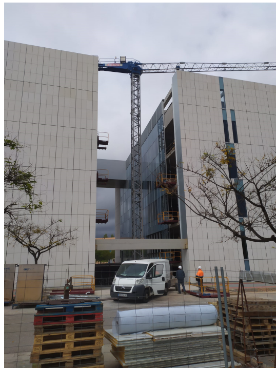
Figure 3.16: Building under construction 3
