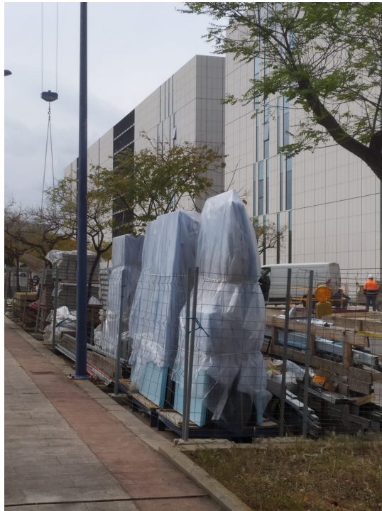
Figure 3.15: Building under construction 2
