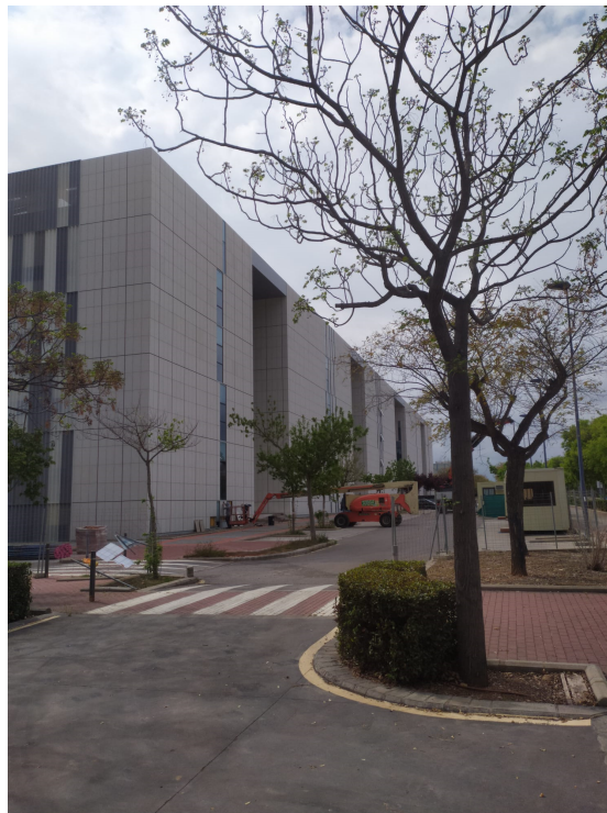
Figure 3.14: Building under construction 1
