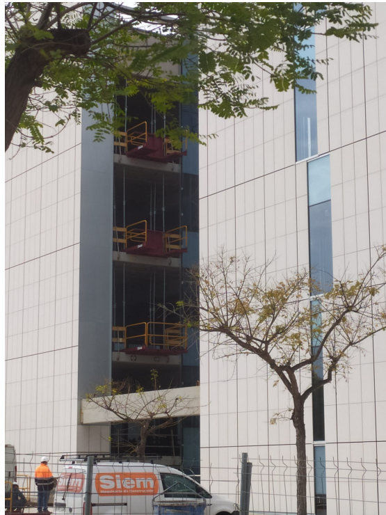
Figure 3.17: Building under construction 4
