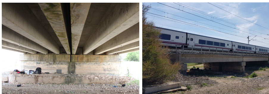
Figure 1: Old Guadiana Bridge: general view.
