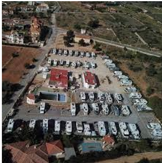
Figure 1. Las Moreras AC Facilities
