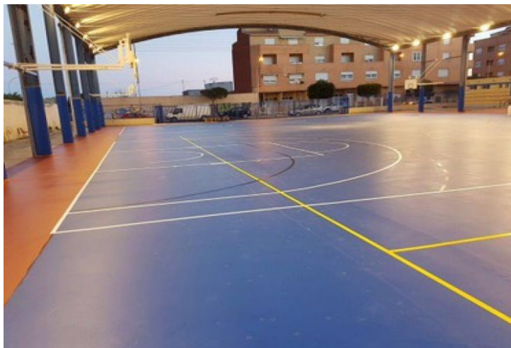
Image 36: Annex pavilion of Benicarló
