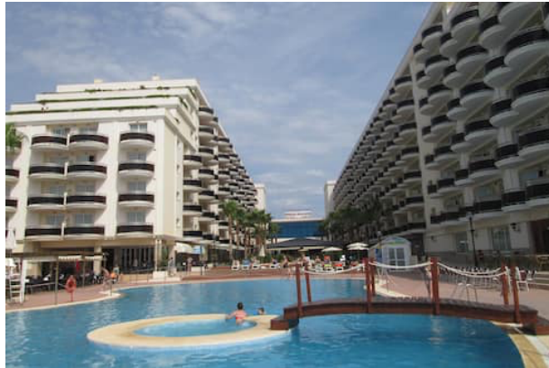
Figure 2. Hotel&Spa Peniscola Plaza Suites
