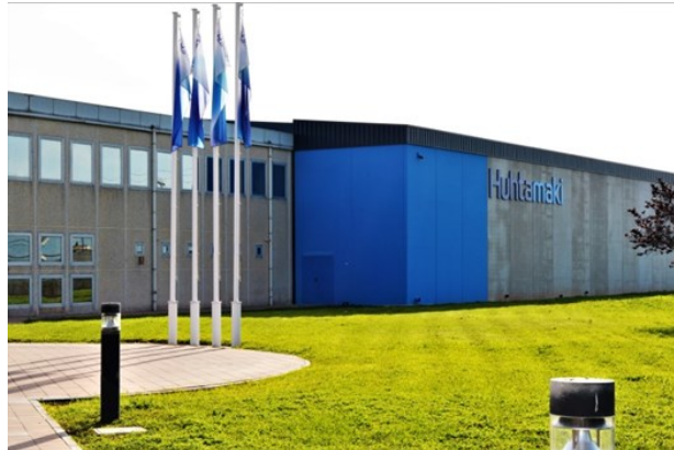
Image 3. Huhtamaki, site in Nules province of Castellón.
