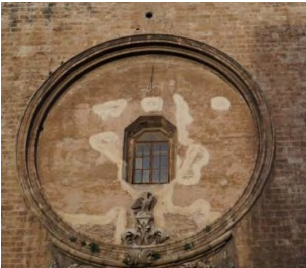
Figure 4. Detail of the “O” of San Juan
