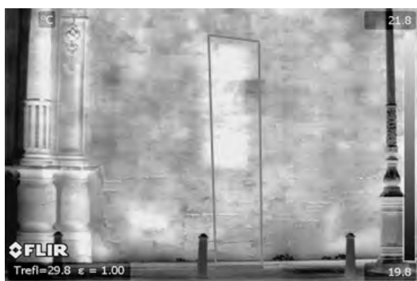
Figure 7. Thermographic image of the San Juan Cemetery façade
