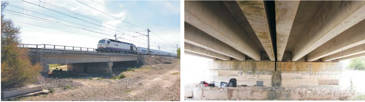
Figure 1: Old Guadiana river bridge.
