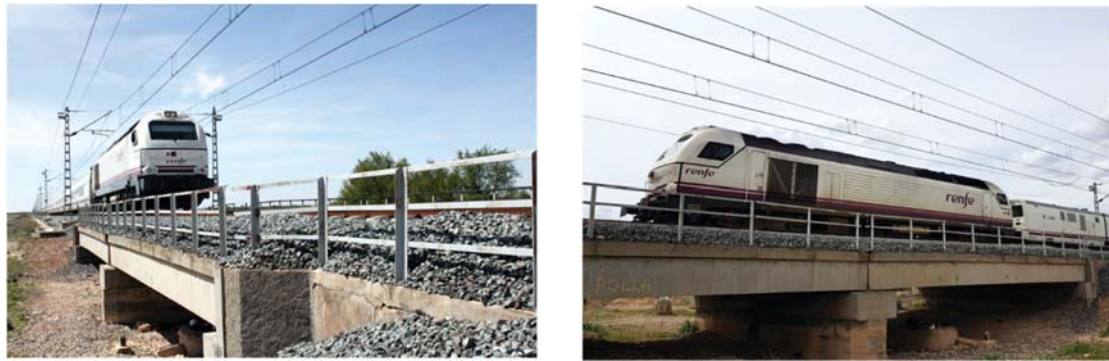
Figure 10: Renfe Altaría Talgo VI trains crossing Old Guediana Bridge.
