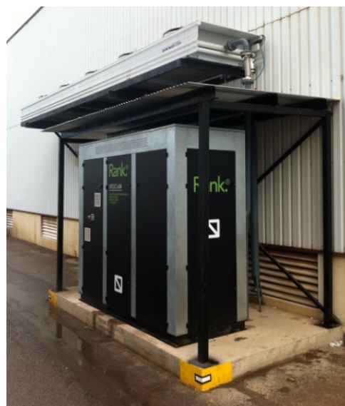
Fig. 4. Rank® ORC HT-20 kWe
