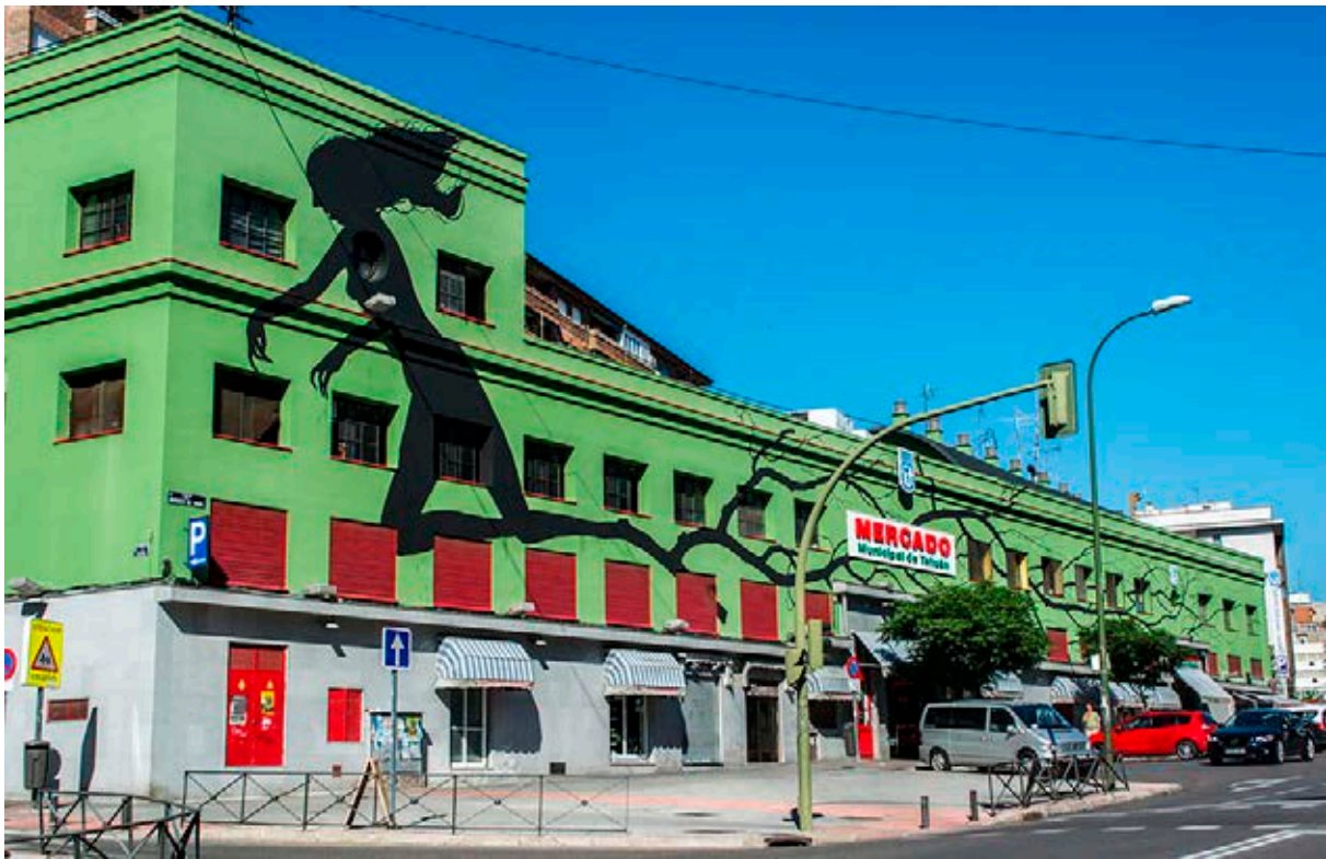
Tetuán Market, painted by David de la Mano and Pablo S. Herrero for Madrid Paisaje Urbano in 2014. Photography: http://porlacalledealcala.blogspot.com.es
