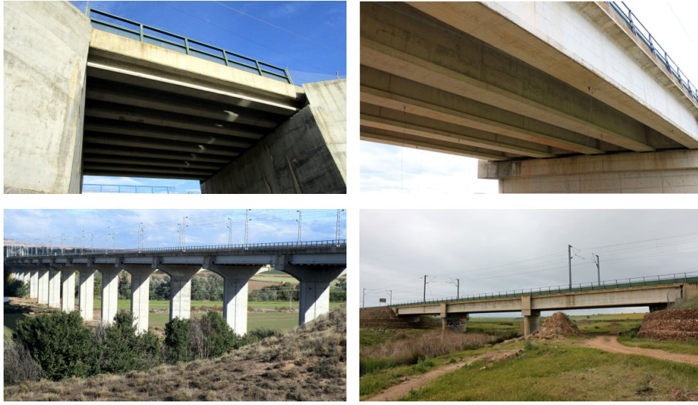
Figure 4: Precast pre-stressed double-T girder decks in Madrid-Sevilla HS line.
