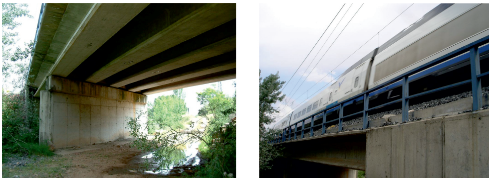
Figure 13: Arroyo Bracea bridge photographs.
