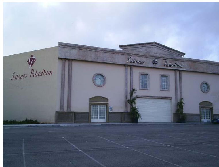
Figure 13: Local Paladium Halls (exterior)
