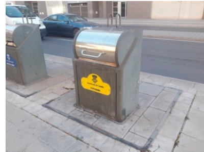
(b) Light packaging underground bin (3 m 3 ). Automatic crane loading.
