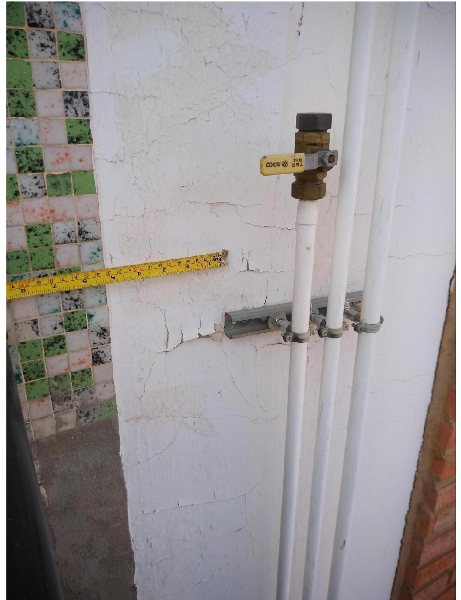
Cimentación y estructura. LS [EH] d_ath01 [Ref. ES002]
