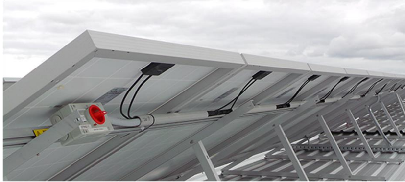
Figura 20. Micro inverter in situ
