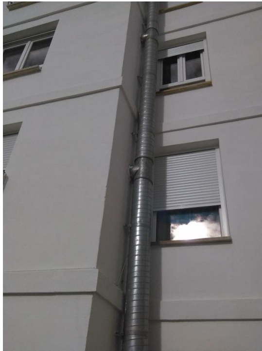
Figure 11. Chimney of the residential block
