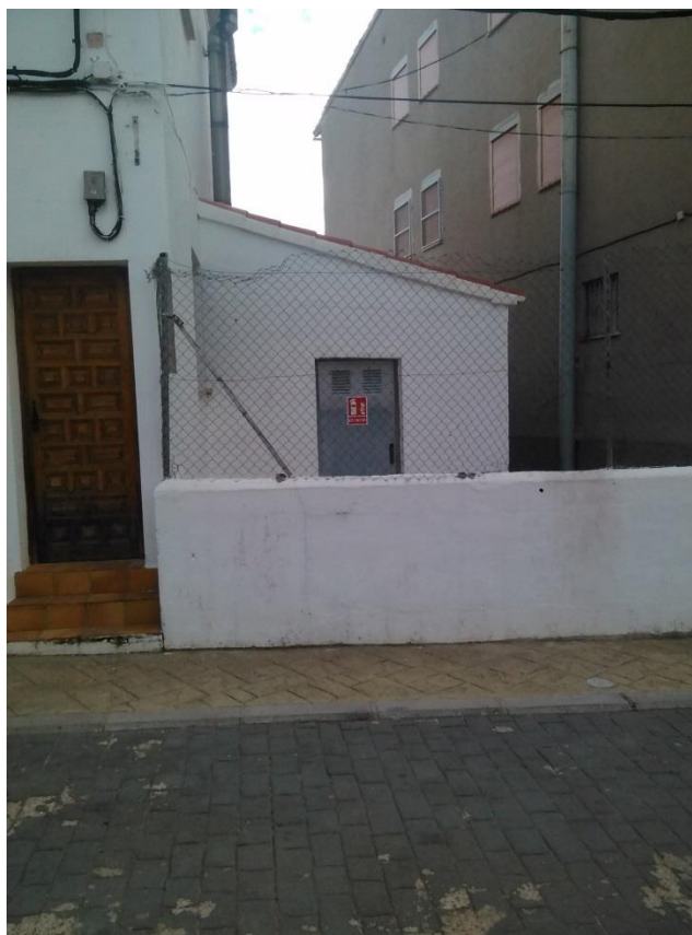
Figure 18. Small house of the school
