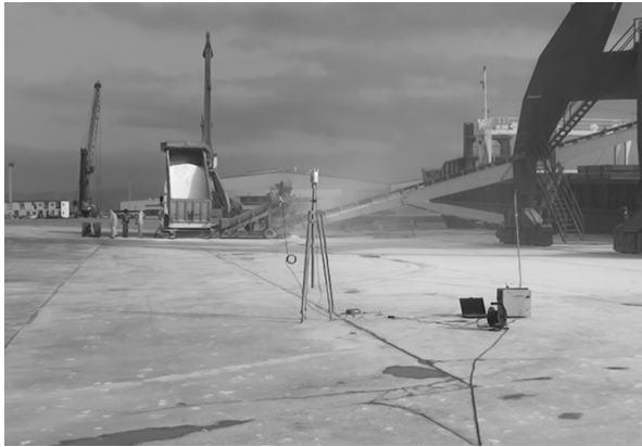
Fig. 4: Truck discharge and conveyor belt transfer.
