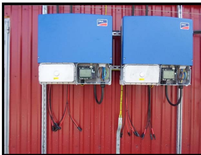
Figure 25. Installed inverters
