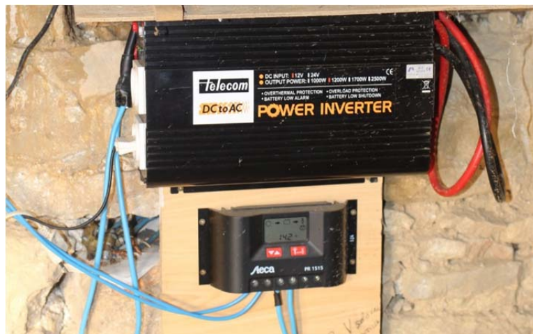
Figure 5. Photovoltaic installation.
