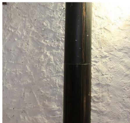
Figure 12. Tube of the chimney.
