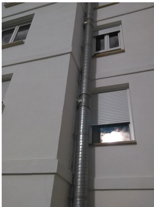
Figure 13. Chimney of the residential block
