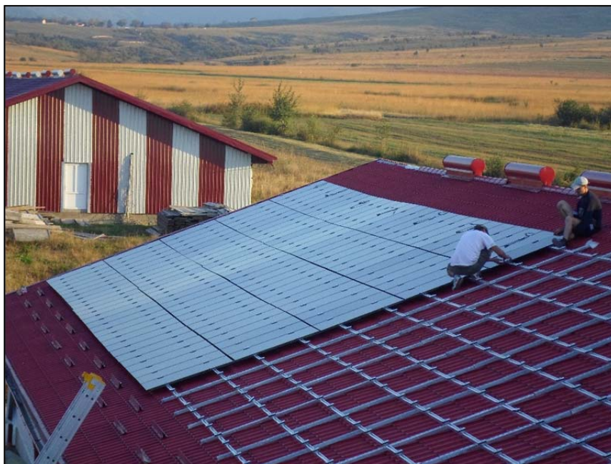
Figure 23. Installing the PV panels
