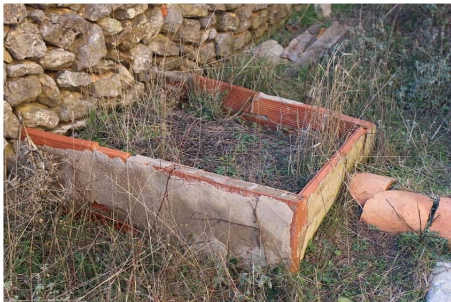
Figure9. Point evacuation of wastewater.
