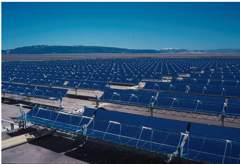
Figure 3. Part of the 354 MW SEGS solar complex in northern San Bernardino County (California), via Wikimedia Commons.
