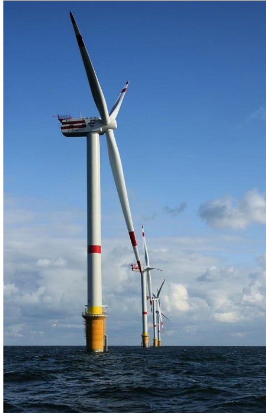
Figure 8. Offshore wind farm, using 5 MW turbines, at Thornton Bank. © Hans Hillewaert, via Wikimedia Commons.
