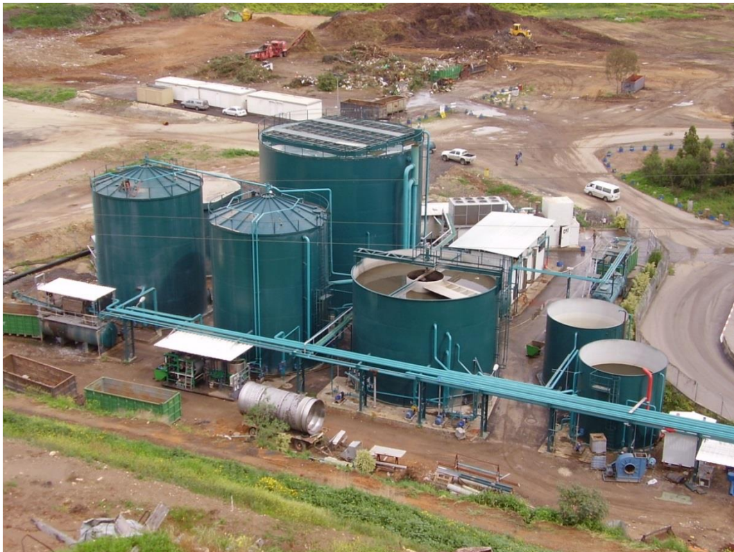
Figure 11. Farm-based maize silage digester located near Neumünster in Germany, by Vortexrealm at English Wikipedia [CC BY-SA 2.5], via Wikimedia Commons.
