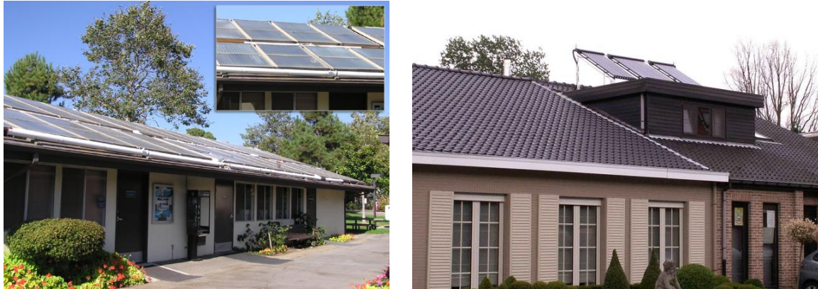
Figure 1. Solar water heating installations, by Alanmak~commonswiki, licensed under CC-BY-SA-3.0, and by KVDP [Public domain], respectively, via Wikimedia Commons,
