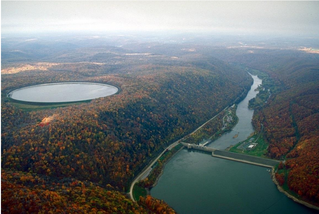
Figure 4. The Seneca Pumped Storage Generating Station reservoir. Source: Wikipedia.
