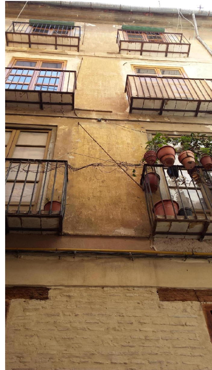
Fachada F1. Acabado exterior [Ref. FA002]
