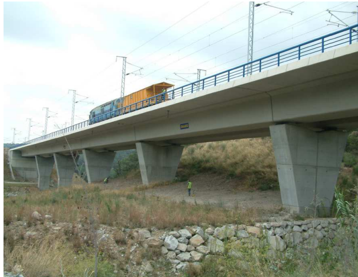
34 Fig. 1. Twin-box girder bridge on Madrid-Barcelona high-speed railway line. Characteristic 35 span length L=30 m
