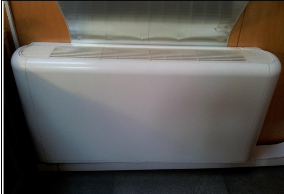
Figura 35: Fan Coil DAIKIN FWV04DATV6V3
