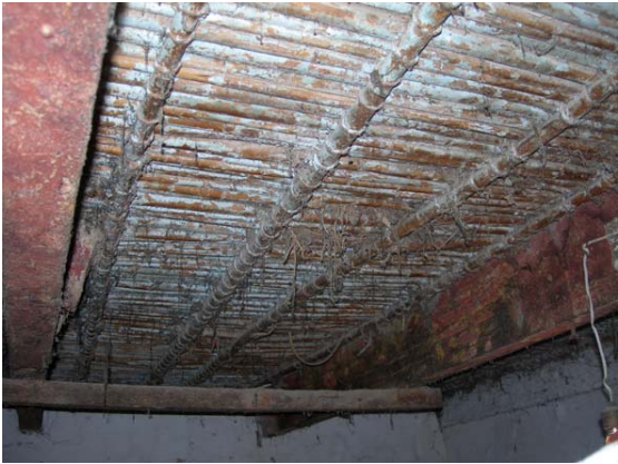
Fig. 11 Reed thatch frame
