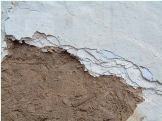
Fig. 12 Adobe wall with numerous coats of lime
