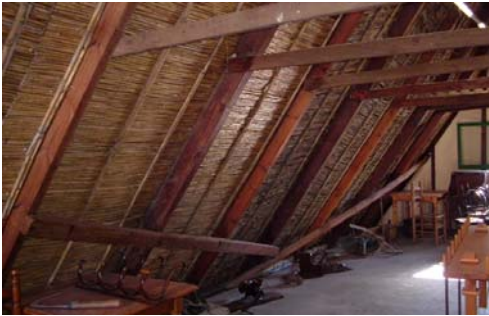
Fig. 10 The andana , space under the roof made with reed thatch frame
