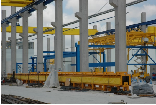
Figura 4.19: Molde de viga rectangular. Ref. PAVI
