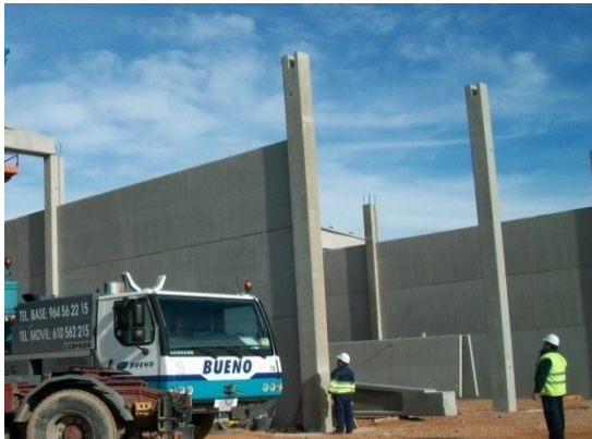
Figura 4.57: Unión galceada, pilar-panel, Ref. PAVI
