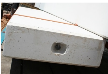
Figura 4.33: Bulones paneles. Ref. PAVI
