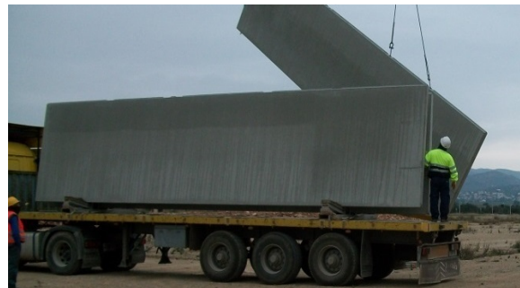
Figura 4.39: Transporte paneles, Ref. PAVI
