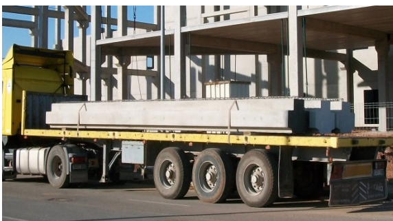
Figura 4.38: Transporte vigas, Ref. PAVI
