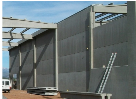
Figura 4.57: Unión galceada, pilar-panel, Ref. PAVI
