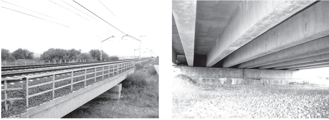
Figure 11: Railway bridge under study
