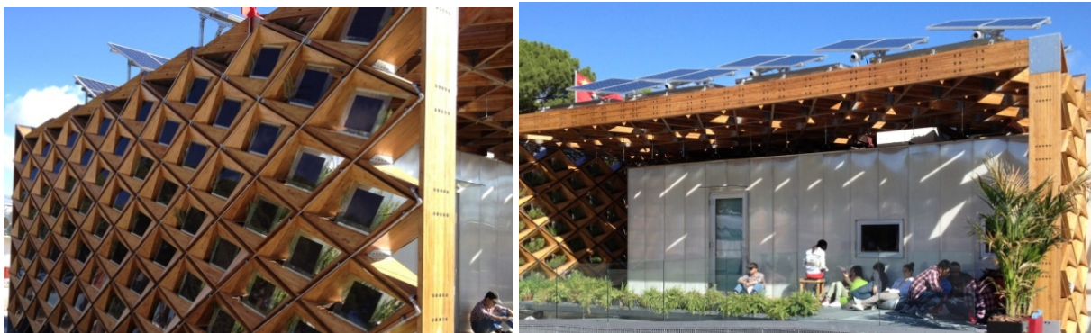
91 Figure 1 The Eco-House prototype exhibited at SDE 2012. BIPV systems are used in the façade and BAPV on the roof.
