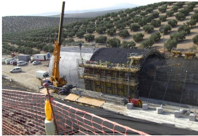
*Imagen 36. Falso túnel (bottom up)*
