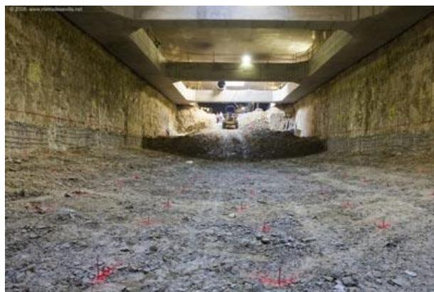
*Imagen 37. Falso túnel (top down)*
