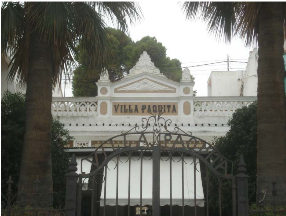
FIGURE 1 Villa Paquita, located along the beachfront promenade, is named in plaster across the front of its façade and on the wrought iron gate to the property.
