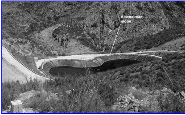
FIG. 9. Leachate dam for a rejects landfill.
