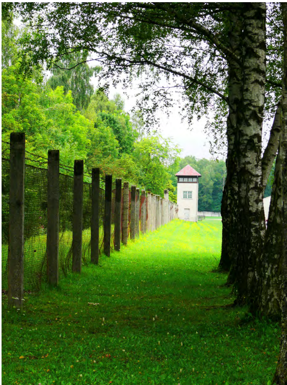
1. Dachau: tanca perimetral
