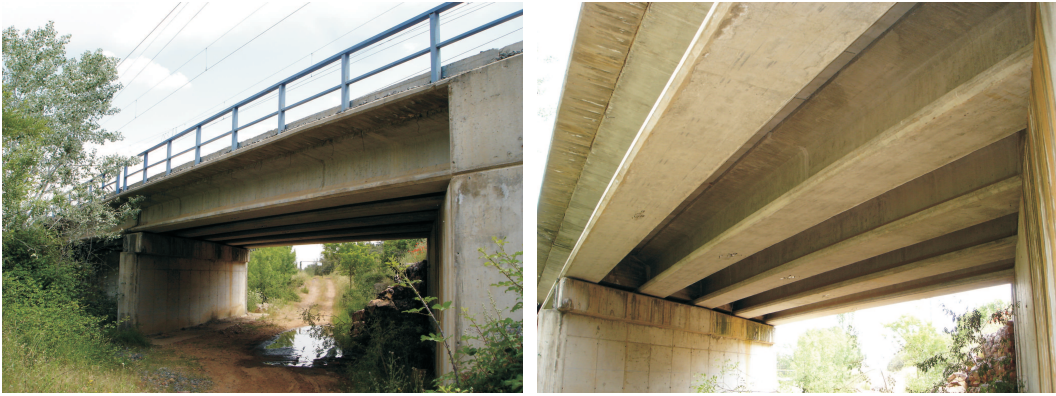
Figure 13: Arroyo Bracea I bridge.
