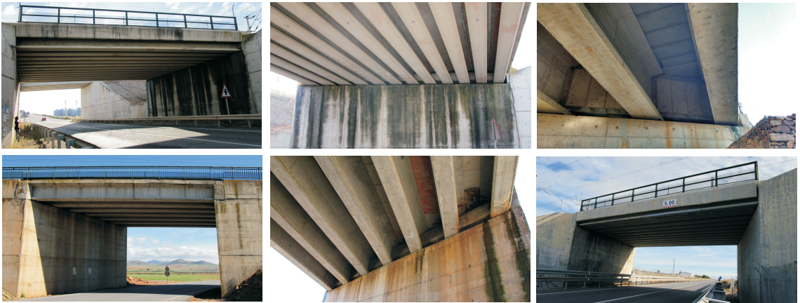
Figure 1: SS girder bridges of the high-speed railway line Madrid-Seville.
