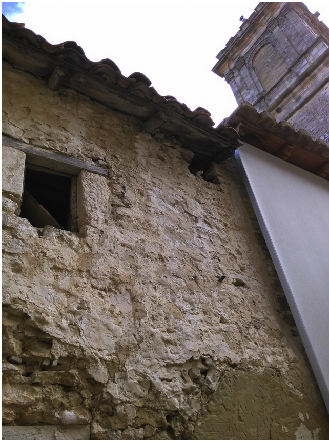
Fig. 1. Example of plundering process of historical coating mortars in Culla (Spain).
