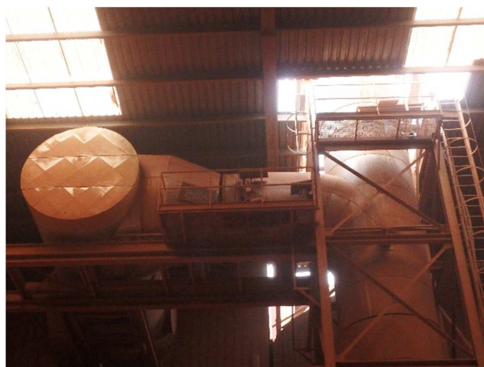
Figura 25. By-pass gases de escape
