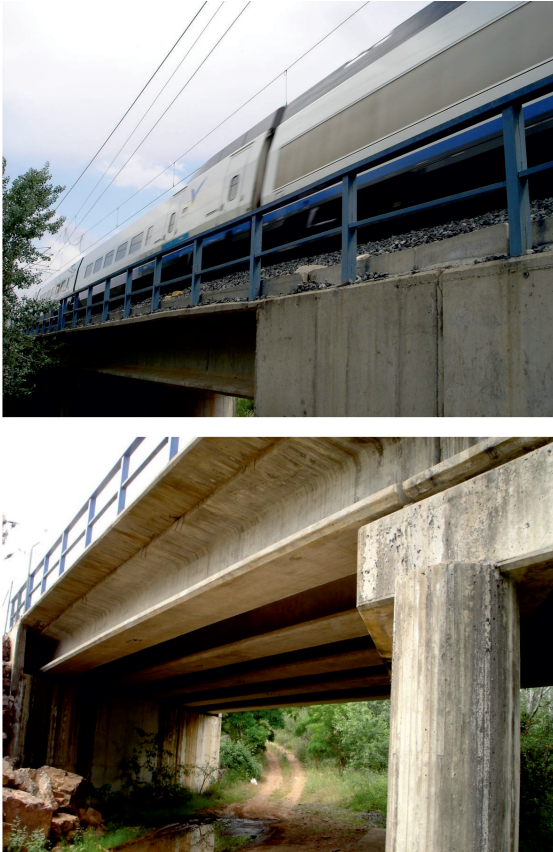
Figure 1: Railway bridge in Spanish high speed line composed by short simply-supported bays
